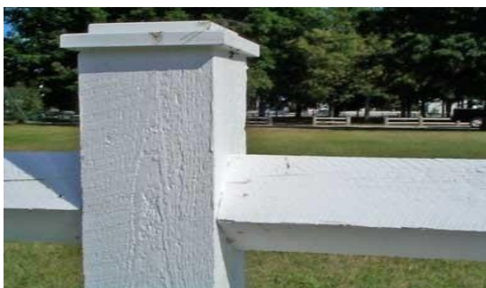
Figure 18. Butt-joint (acceptable)
