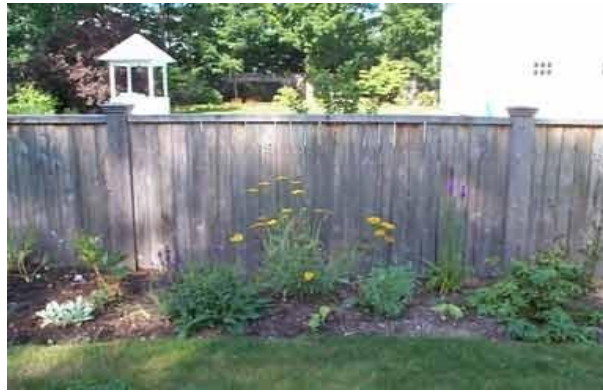
Figure 13. Four (4) foot solid board fence with molded caps and post caps enclosing a swimming pool and spa
