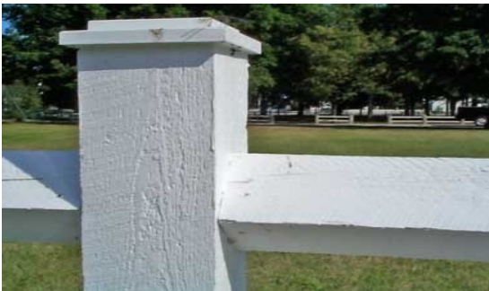
Figure 18. Butt-joint (acceptable)
