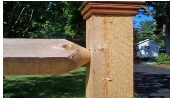
Figure 19. Dowel Joint (not acceptable)
