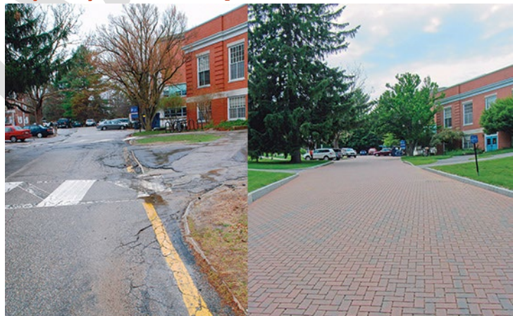
Figure 42 Before and after application of interlocking pavers on a roadway at the University of New Hampshire
