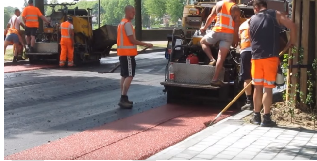
Figure 19 Hot-mix terra cotta asphalt colorant
