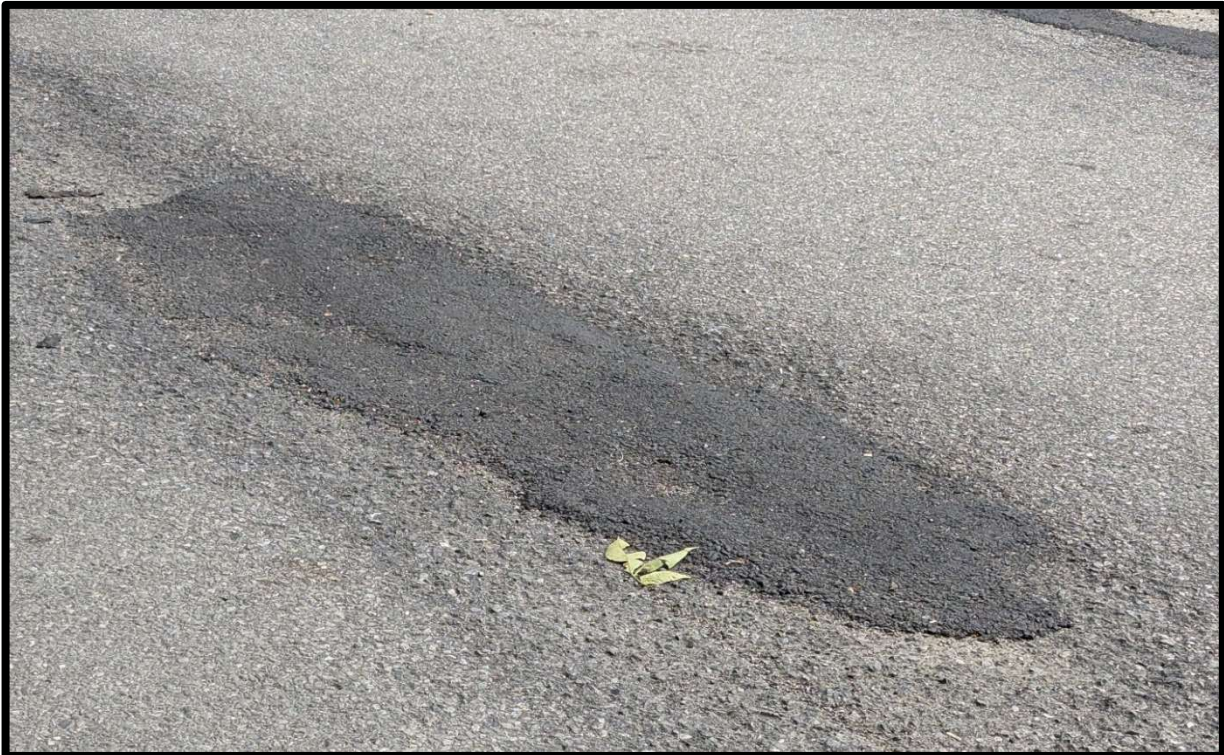
Photo 2: Christian Hill Road – Previously patched center line cracking
