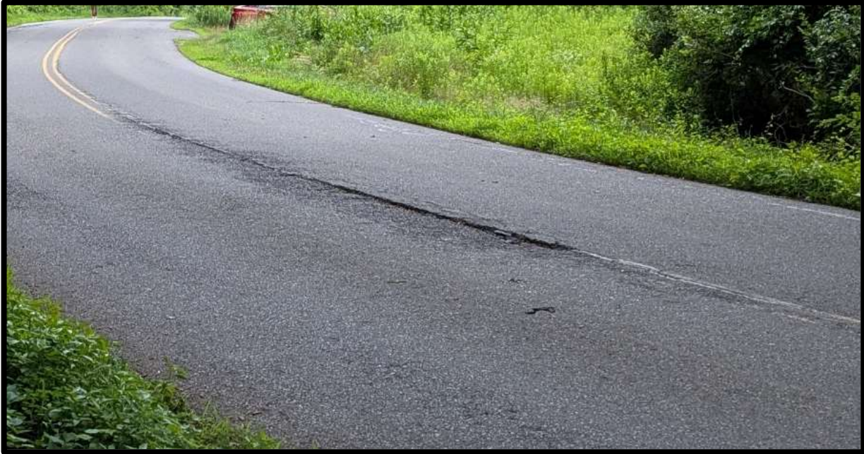
Photo 1: Christian Hill Road – Existing cracking at center line
