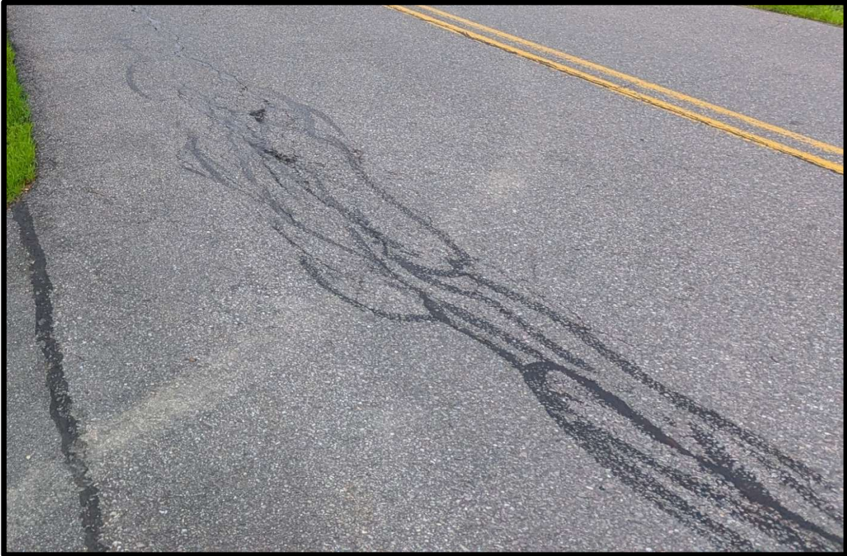
Photo 3: Christian Hill Road – Previously sealed cracking
