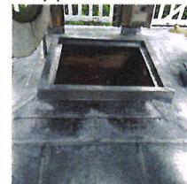
Lead Coated Copper Flat Roof
