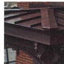
Standing Seam Metal Roof
