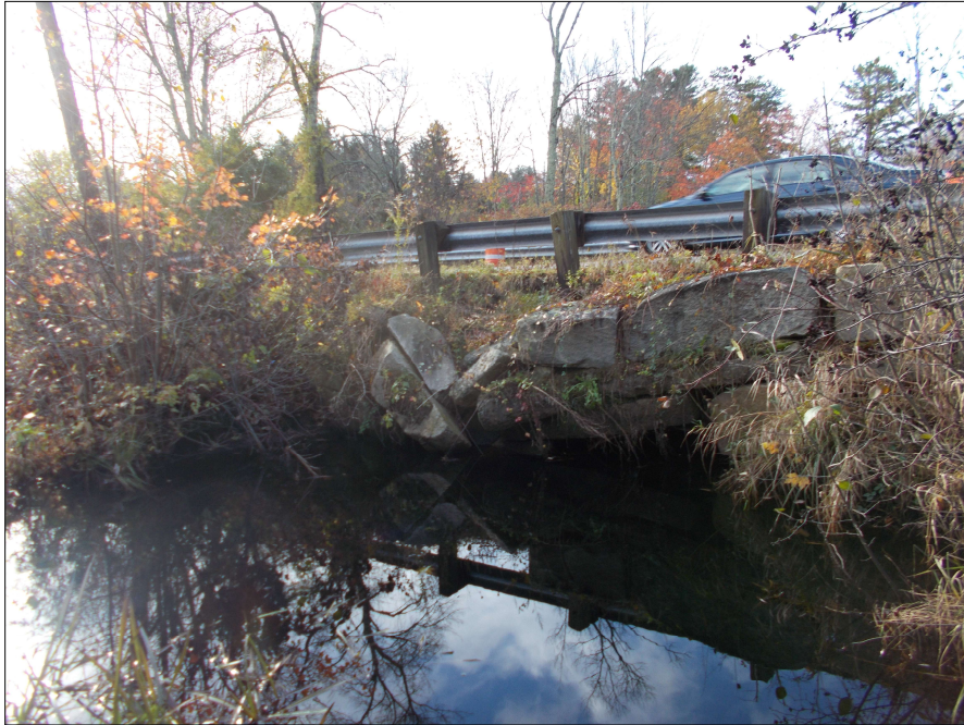
Collapsed Upstream Headwall
