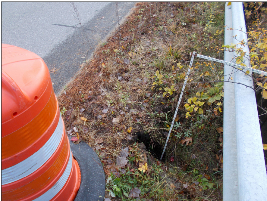
Sinkhole at Downstream Headwall
