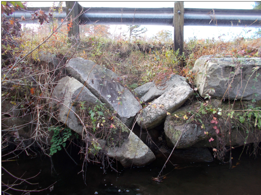
Collapsed Upstream Headwall
