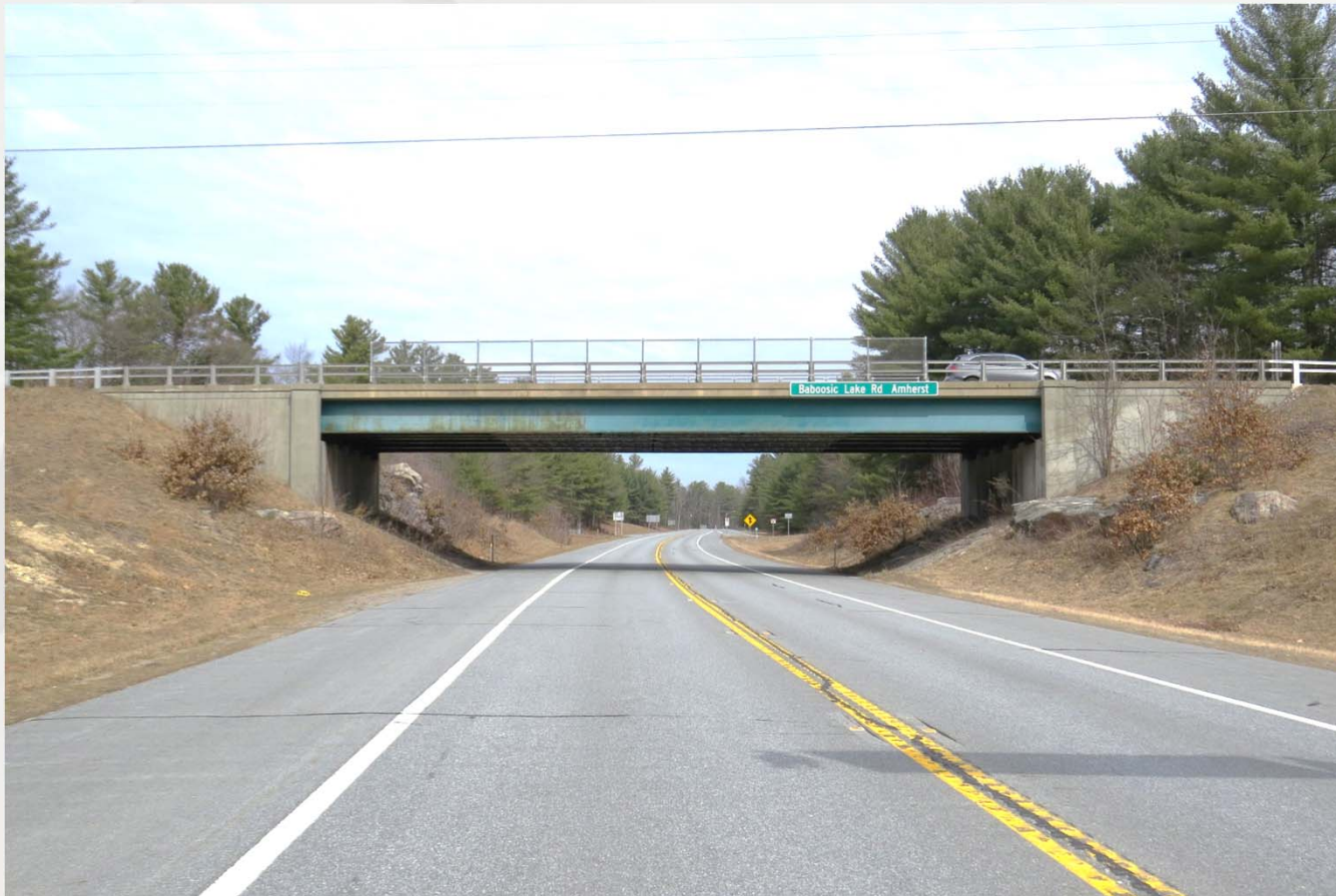
Bridge Elevation Looking North (East on NH 101)
