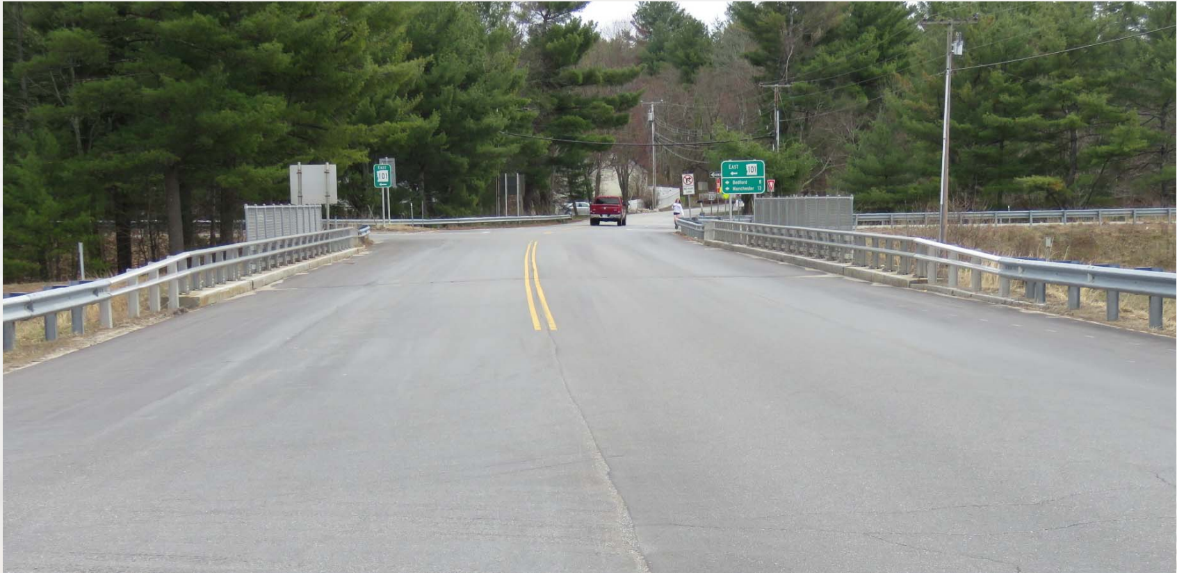
NH 122 - Looking East Across Bridge
