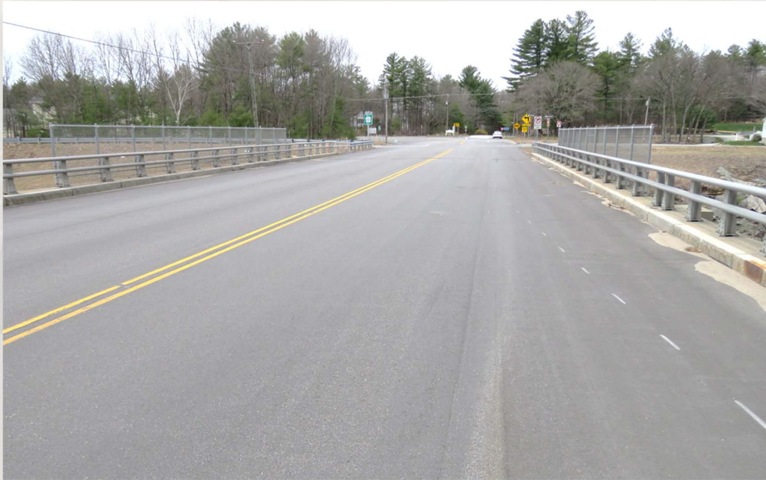
NH 122 - Looking West Across Bridge
