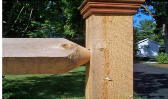
Dowel Joint (not acceptable)
