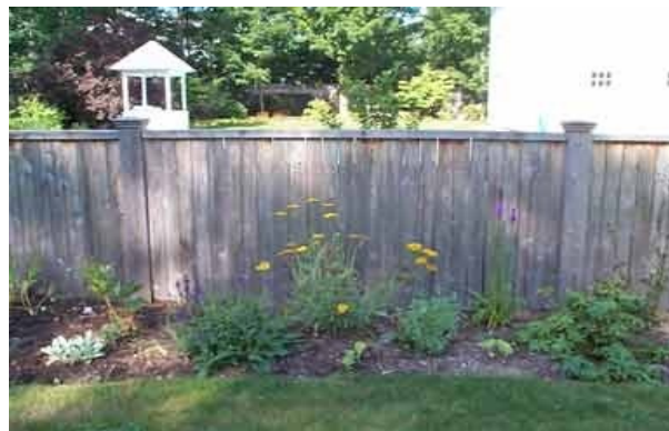
Four (4) foot solid board fence with molded caps and post caps enclosing a swimming pool and spa.
