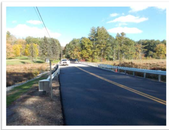
Completed Horace Greeley Road
