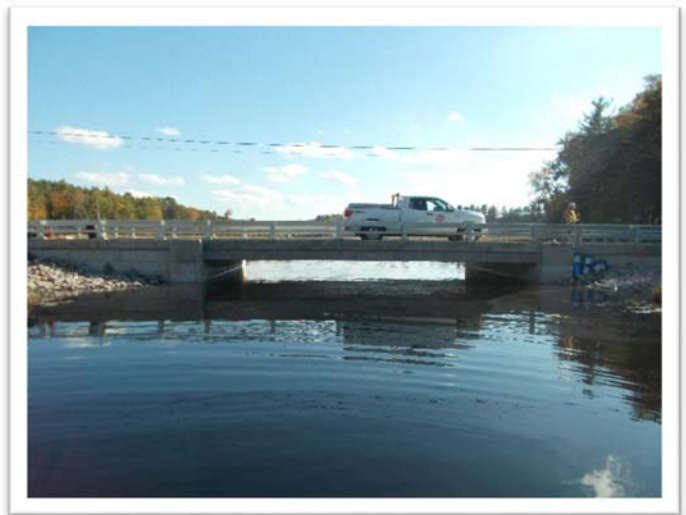
Upstream Elevation of the Completed Bridge
