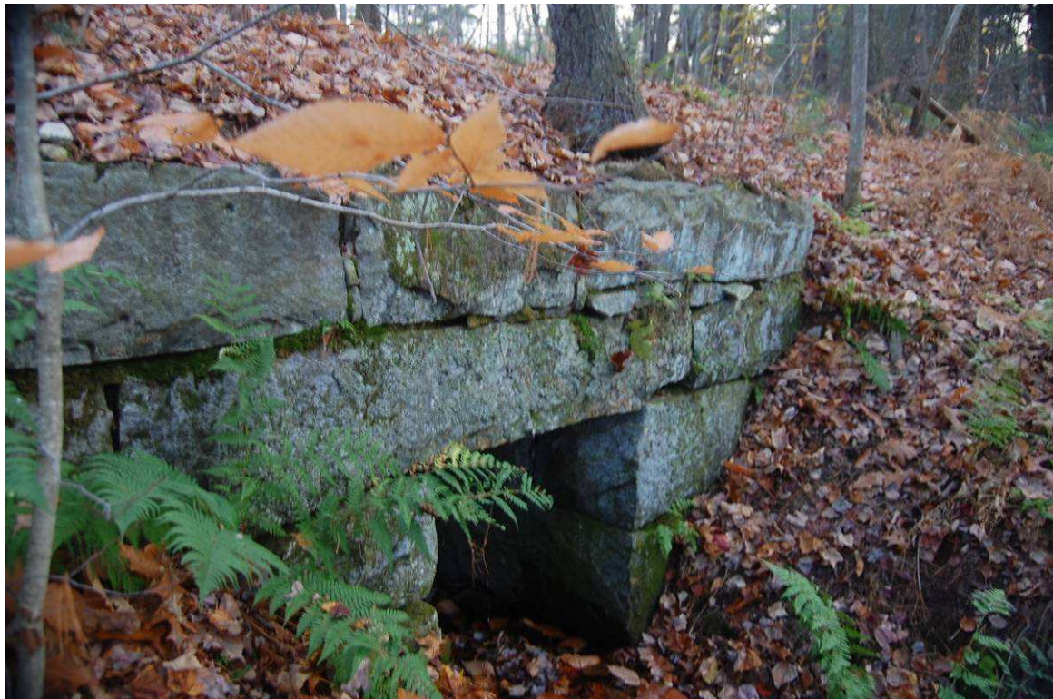
Photo 88 description: Granite box culvert between Walnut Hill Road and Dream Lake for Manchester & Milford (#226)
