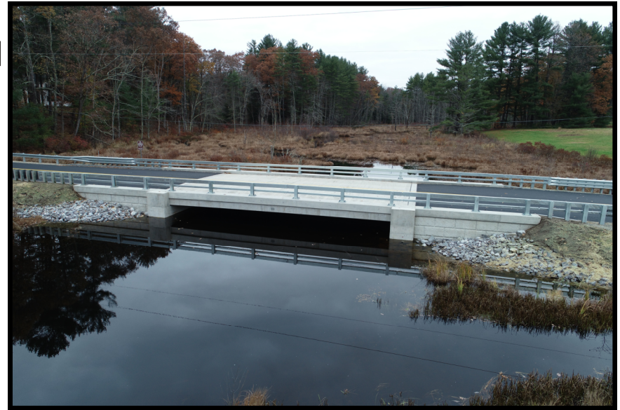
Precast Prestressed Concrete Deck Beam Bridge Horace Greeley Rd., Amherst, NH November 2018
