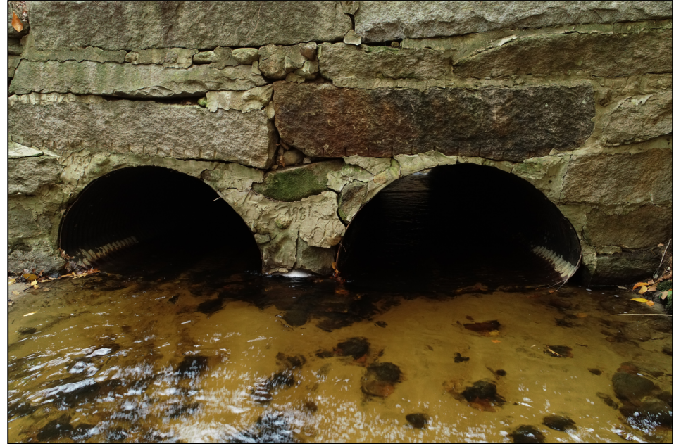
Closer View of Deterioration with Missing Mortar, Stones Shifting, Corrosion, and Undermining of CMPs
