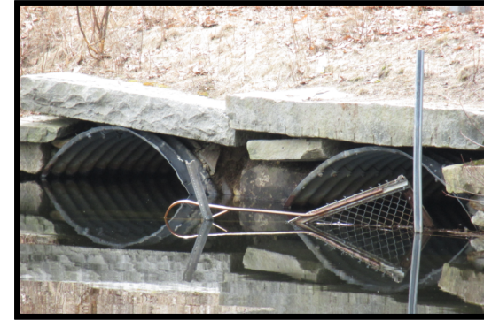
Collapsed Headwall
