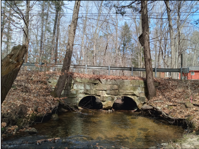
Downstream Headwall Undercutting of Banks Visible
