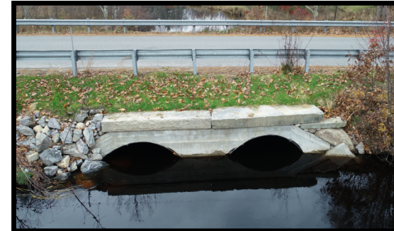
Repaired Headwall
